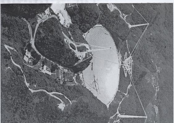
Fig. 4.6. The 305-m spherical radio dish at Arecibo in Puerto Rico. The instruments at the prime focus feed, suspended from three tall pylons. (The Arecibo Observatory is part of the National Astronomy and Ionosphere Center, which is operated by Cornell University under a cooperative agreement with the National Science Foundation.)
